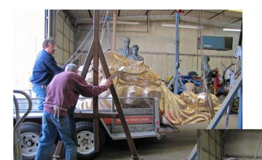
• The sculpture was lifted off the trailer with gantries and lowered onto heavy paper to make a template for locating the sculpture and the mounting holes on the base during installation.
