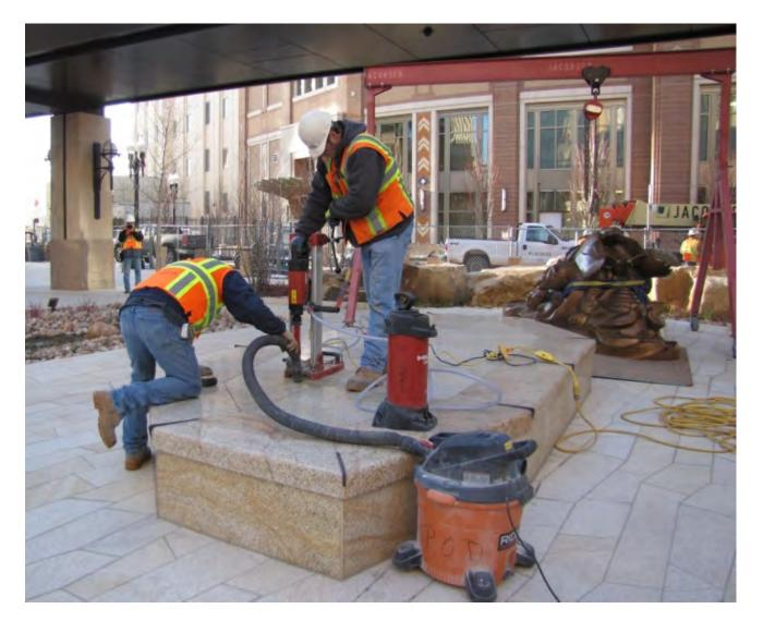
With the sculpture suspended over the base and the mounting pegs inserted, the holes are dried of the water used as coolant during the drilling and epoxy is then inserted into the holes.
